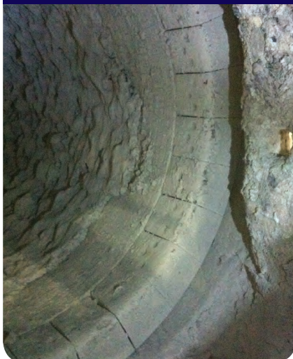
Figure 6: SIFCA nose blocks in a \phi 4.3m precalciner kiln producing 3200tpd of clinker, after one year of service
