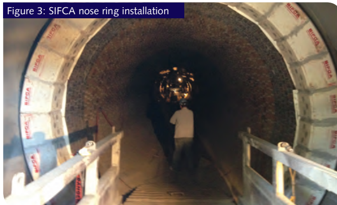
Figure 3: SIFCA nose ring installation
